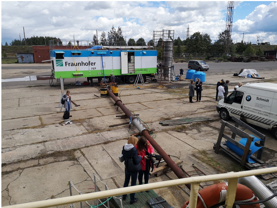
The connecting pipe and the accelerator on truck. (Image: ARIES)
