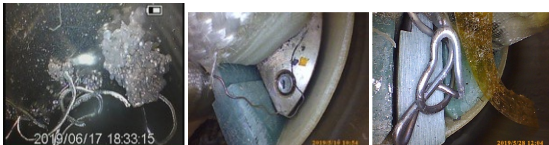
Figure 11. Examples of the debris removed during the cleaning process.
