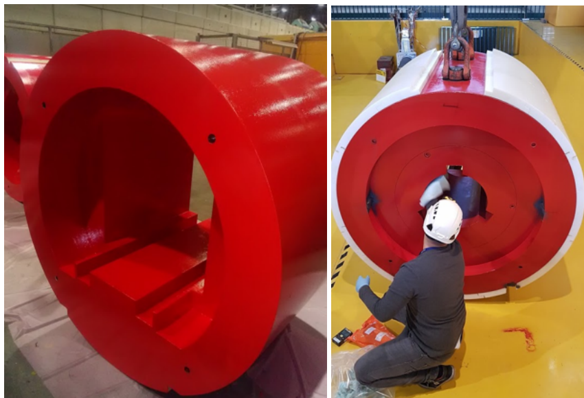
Figure 49. Left: view of the new JTT shielding before installation of the borated polyethylene plates. Right, the old JTT after removal. Note the small cylindrical opening vs. the new square shape and the slots for the supports of the VT chamber in both pieces.
