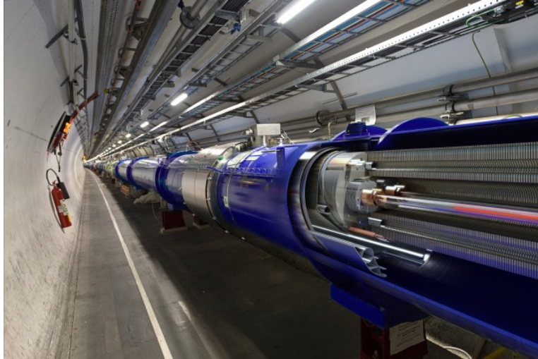
Fig. 2) 3D cut of the LHC dipole Image Credit: CERN
