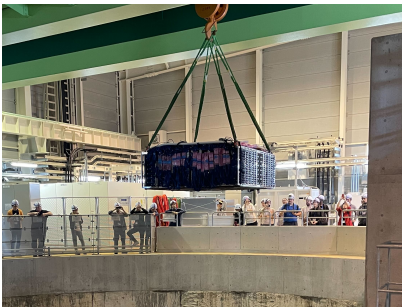
(iv) Installing the detector into the pit by a crane
