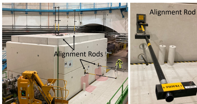
FIG. 20. Alignment rods installed during inspection.
