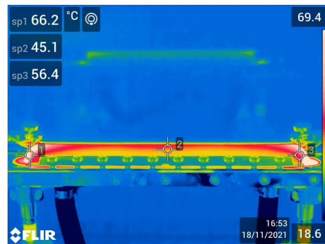
Figure 4: Lateral view picture taken with a FLIR E75 IR camera thermal measurements for in-air testing with 150 A injected in the 1 mm wire. All screws clamping the insulator in place have a 1 N m torque
