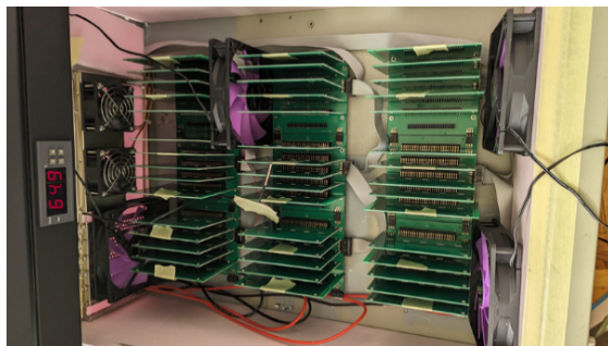
Figure 6. ESS box for 45 VFE and 9 LVR cards with ventilators for ambient air exchange (left) as well as ventilators for internal air steering. Stable temperatures of 70 \pm 1.5^\circ\text{C} were achieved.
