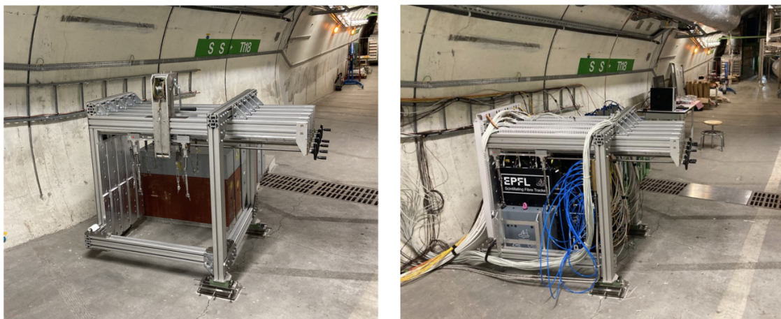
Figure 14. Mechanical support of the target system after the installation (left) and fully loaded with wall boxes and SciFi planes (right).
