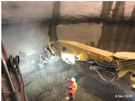
Fig. 6. Excavator with hydraulic cutting heads being used at HL-LHC Point 1.
