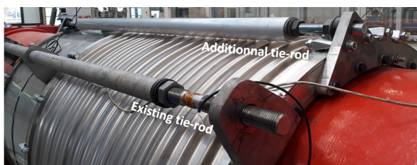
Figure 7: Prototype of additional tie-rod (autumn 2019).
