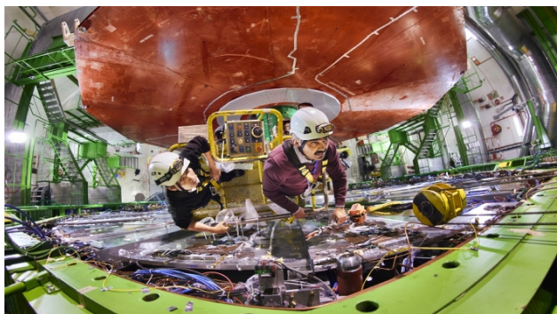
Figure 2. A picture taken during the removal of one of the RE+4 supermodules.
