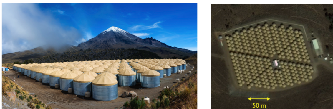
Fig. 11: Views of the HAWC array of water tanks. Left: ground view (J. Goodman, 2016). Right: satellite view; at the centre is the Counting House with the electronics and computing; on the right is the HAWC Utility Building with the water filtration plant (Google Earth, 2016).
