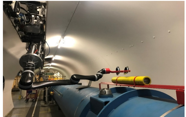
Figure 3: Irradiation source installed on the TIM for BLM validation.
