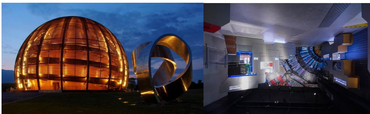
Figure 8: The Globe of Science and Innovation (left) and the Microcosm exhibition (right) at CERN.
