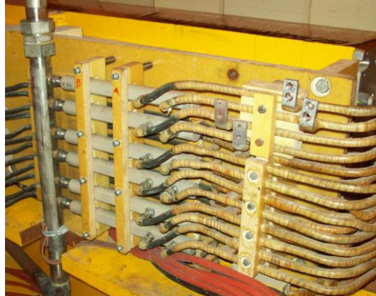
Figure 42: Area where the electric and cooling circuits are split
