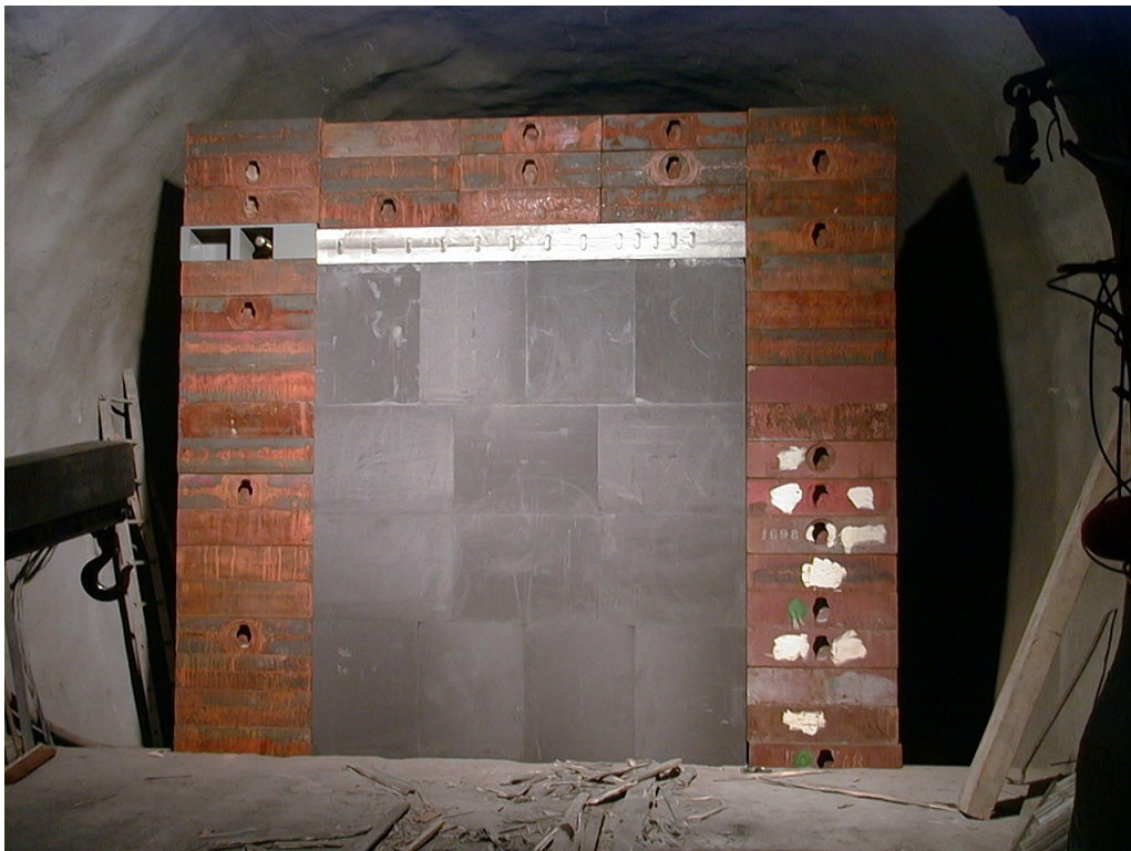
Figure 4.87: View of the CNGS Hadron Stop. Graphite blocks, aluminium cooling plates and CERN Standard Iron blocks are shown.
