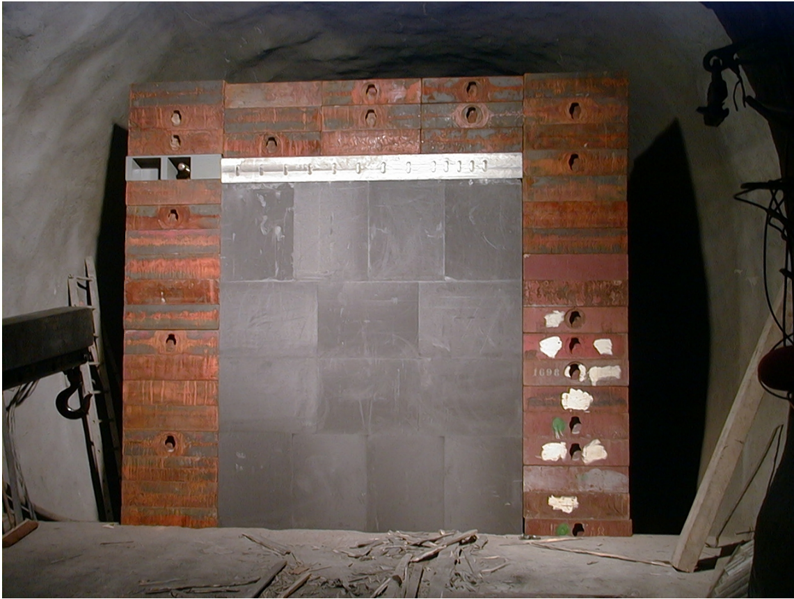
Figure 4.8: The hadron stop during its construction.
