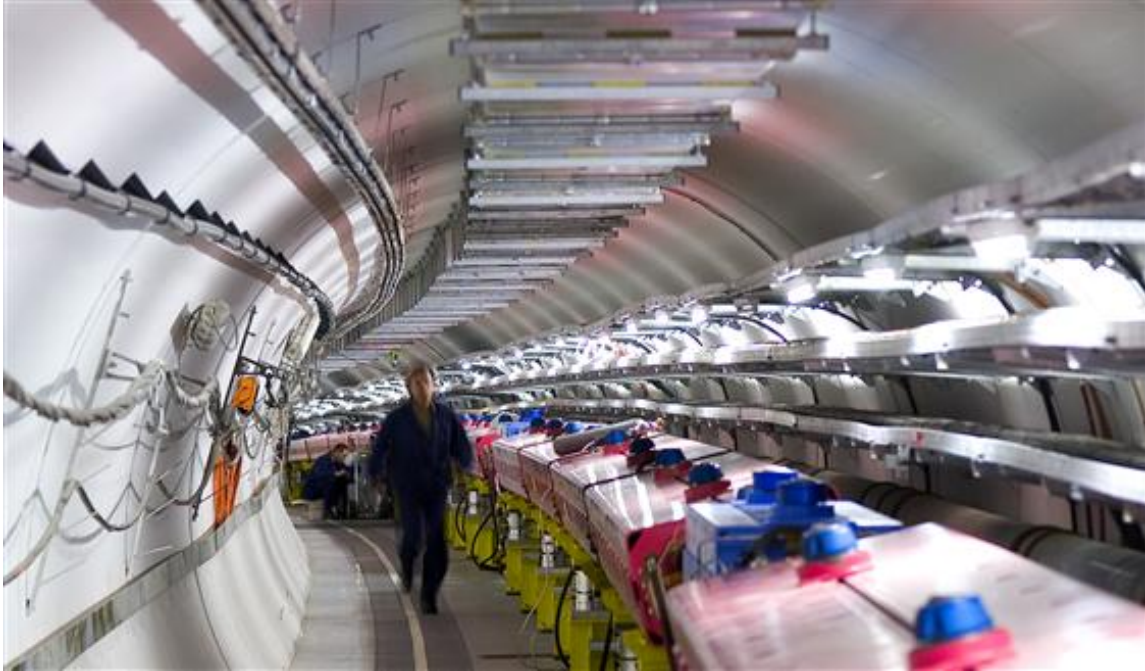
Figure 4.3: Photo of the 800 m proton beam transfer line for CNGS with the tilted magnets.
