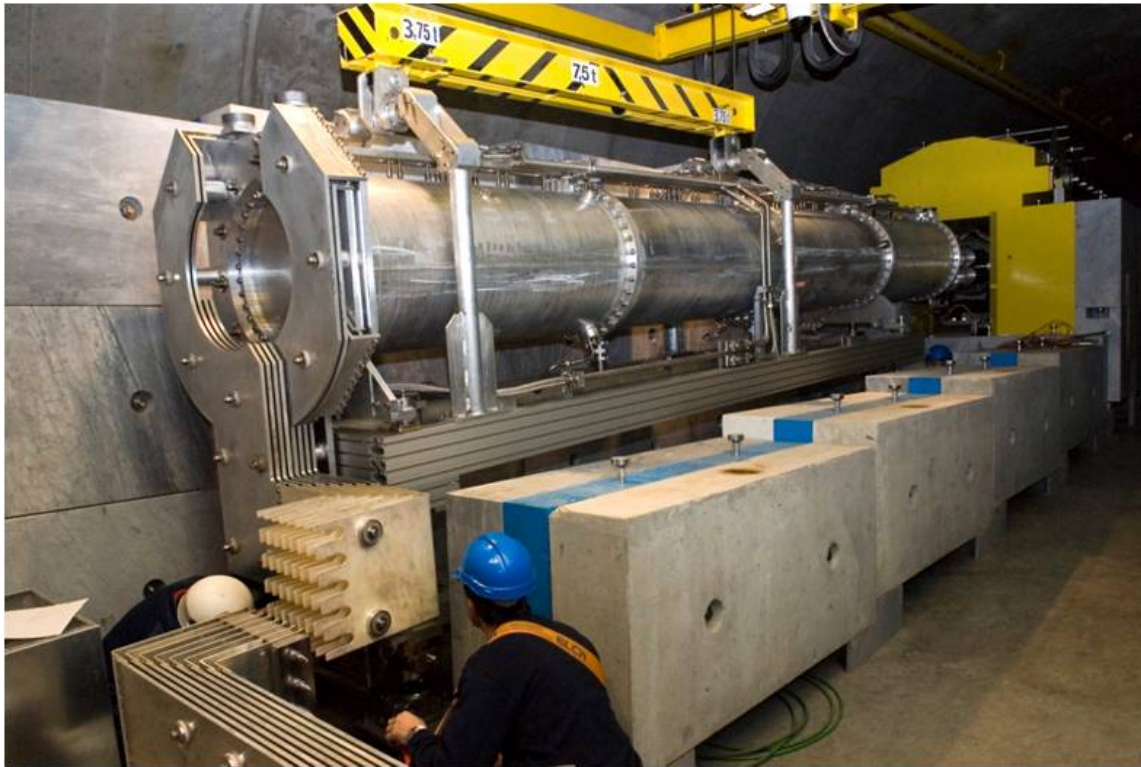
Figure 4.7: Photo of the horn during its installation in the tunnel.
