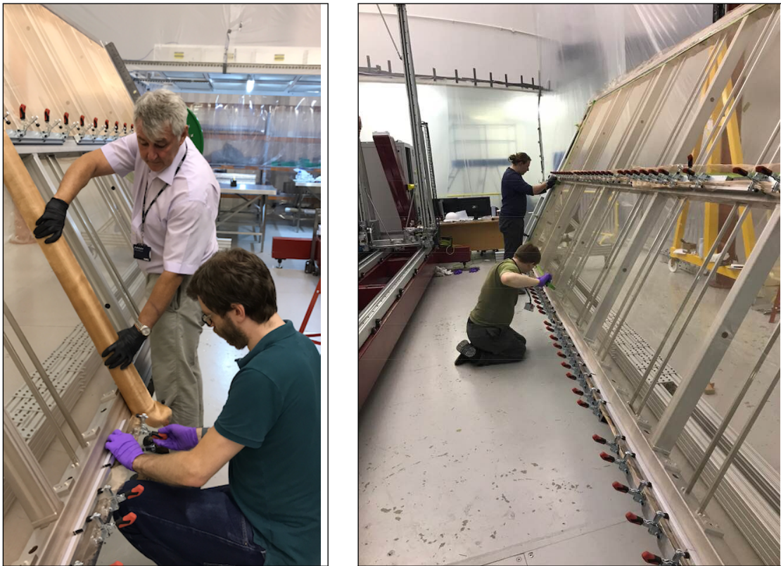
Figure 2.10: Grounding mesh being clamped to the APA and taped off, ready for gluing to a ProtoDUNE-SP frame.
