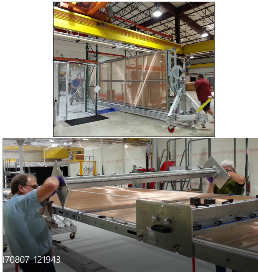
Figure 2.19: (Left) APA being moved around a production facility on the process cart. (Right) APA frame with the grounding mesh already installed is shown sitting on a process cart. Two technicians are using a custom jig to place the wire combs above a horizontal cross beam on the APA.
