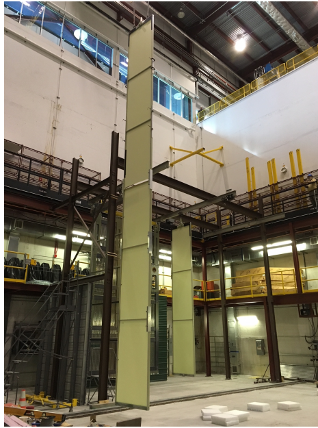
Figure 4.14: A 12 m DUNE-SP CPA mockup panel and a smaller 6 m ProtoDUNE-SP panel mockup at Ash River.
