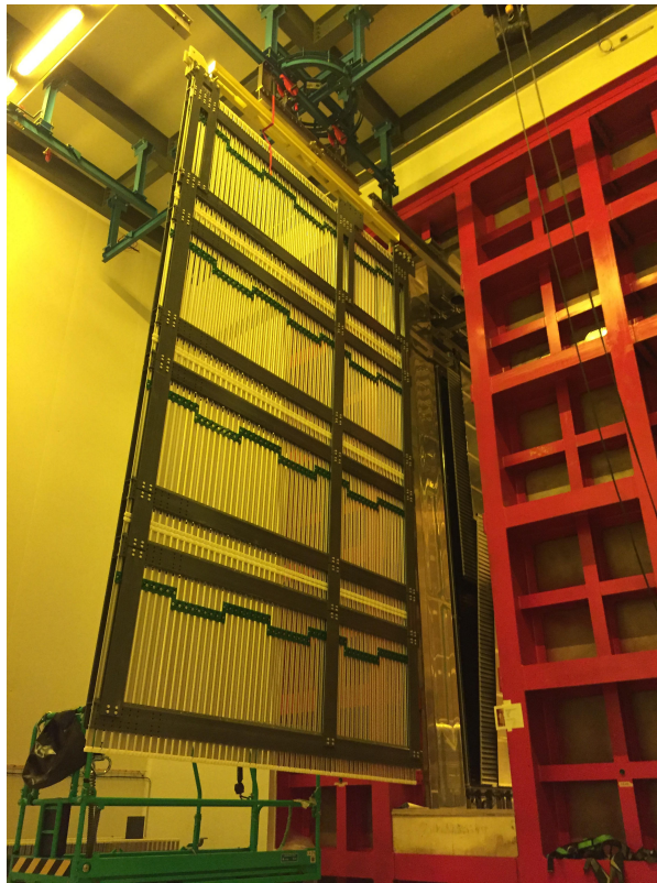
Figure 4.19: Completed endwall in process of installation into ProtoDUNE-SP cryostat.
