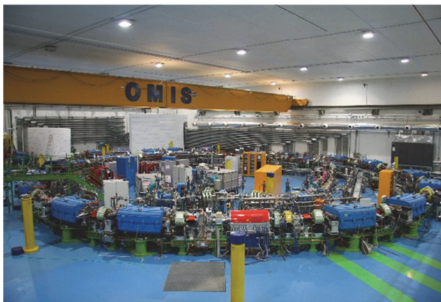
Fig. 10.3. The CNAO synchrotron providing protons up to 250 MeV and carbon ions up to 400 MeV/u with its injector inside the ring (courtesy CNAO).
