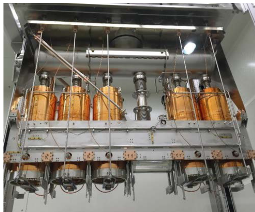
Figure 1: Cavities installed on the cryo-module frame in the cleanroom ISO 5.
