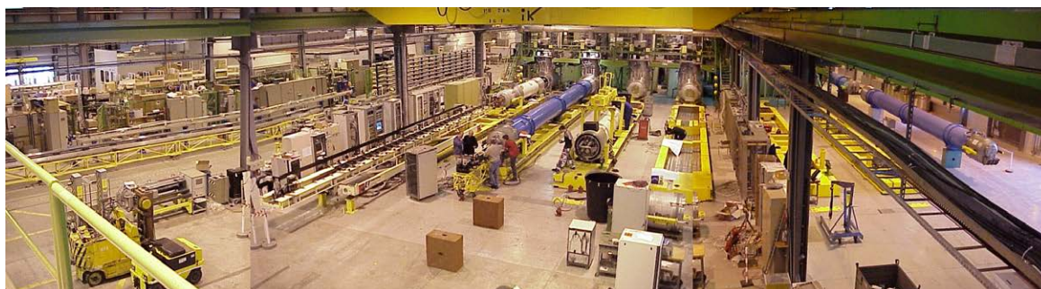
Overview of CERN's Large Magnet Hall (Image Credit@CERN)
