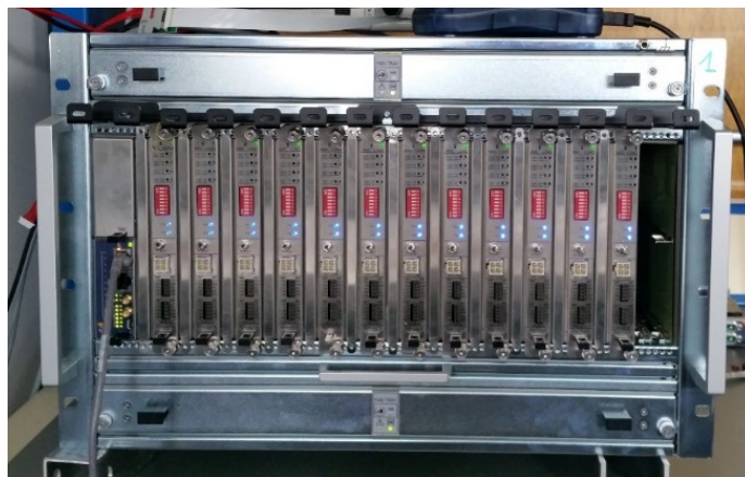
Figure 1. Custom MTCA shelf with AMC load boards.
