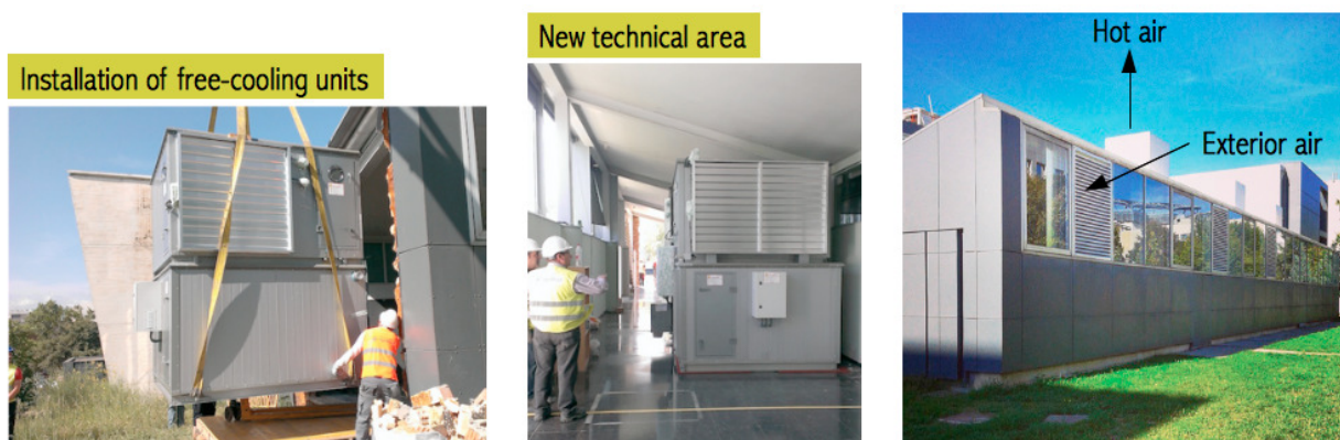
Figure 3. Free-cooling units being installed in PIC, in mid June 2014.
