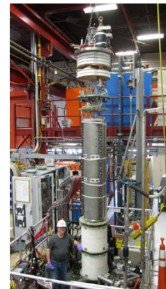
Figure 2: QXF mirror entering the FNAL test station
