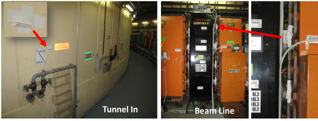
Fig. 9. Location of the passive dosimeters near the PSB beam line and the inner tunnel wall.
