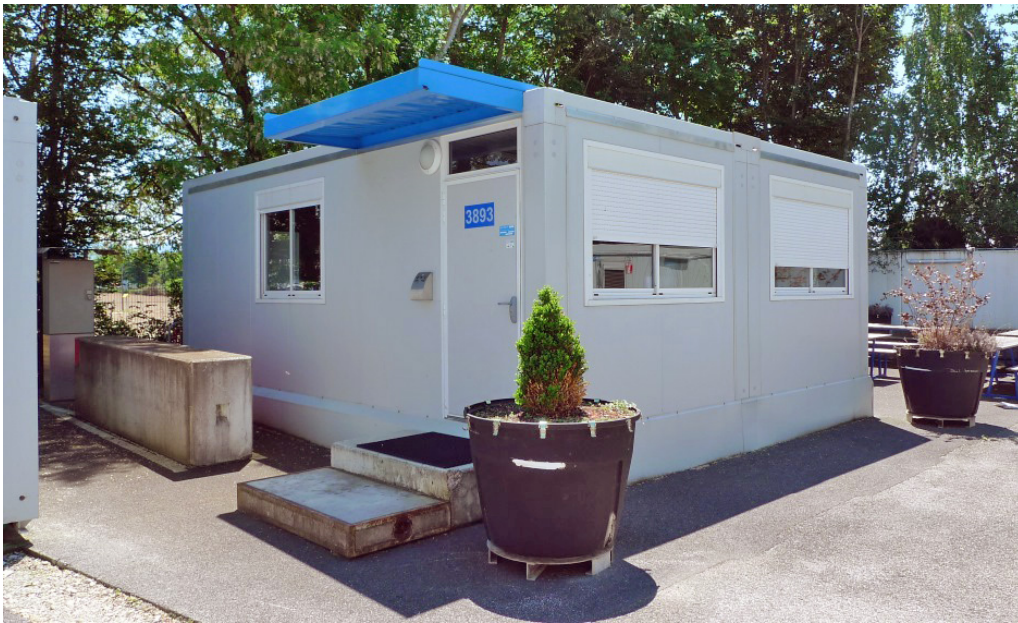
Fig. 9: Example of a meeting room/open office suitable for the CLOUD collaboration. The photograph shows bat. 3893, made from two pre-fabricated units (full dimensions 6 \times 7.5 \text{ m}^2 ) at the LHCb site (LHC Point 8). A similar office, located near the T11 experimental zone, would be suitable for CLOUD.
