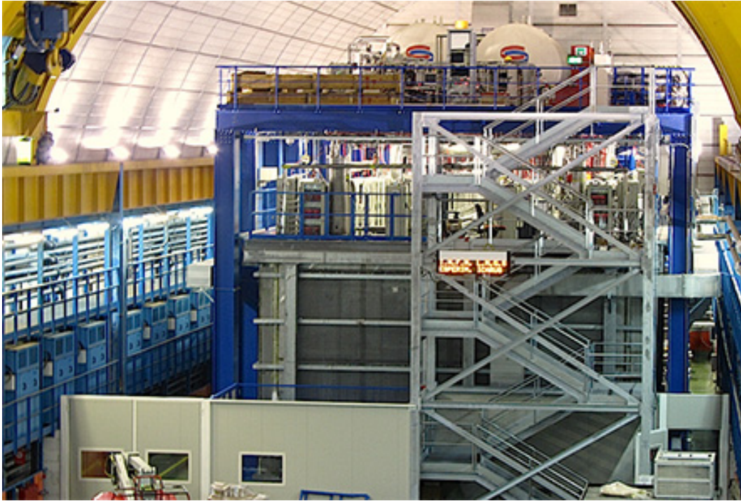
Figure 1. The ICARUS T600 plant in the Northern side of the Hall B at LNGS. Ladders to access the intermediate and the top levels are visible in the front together with the 3 m high wall that separates the T600 area from the rest of Hall B. Cabinets with the readout electronics are visible at the intermediate level. At the top level, the two 30 m 3 cryogenic storage tanks and some additional electronic equipments (HV supply, PMT electronics, trigger system, etc.) are also visible. Most of the cryogenic equipment (nitrogen and argon pumps, cryo-coolers, etc.) is located on the rear side of the T600, at the Northern end of the Hall B.
