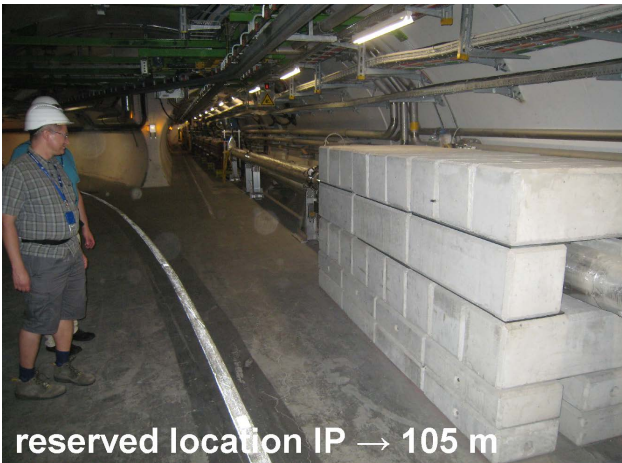
Figure 48: Concrete shielding block installed in the LHC tunnel close to the reserved wire-compensator location [photo R. Steinhagen].
