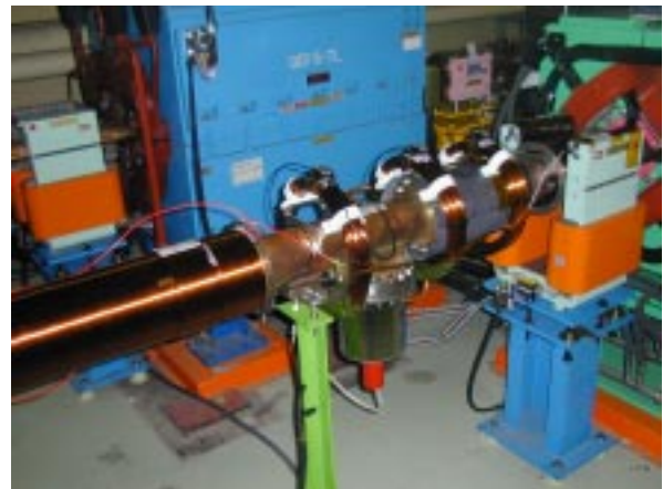
Figure 1: Solenoids in the LER tunnel. The three solenoids on the right side are those installed in bellows-NEG pump sections. The long solenoid on the left side was installed in the first installation.
