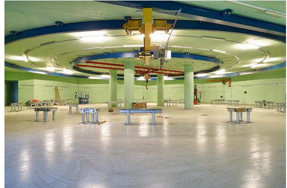
Figure 2: Synchrotron hall with first supports and girders installed
