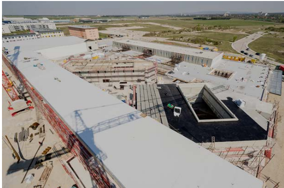
Figure 1: Current status of the building construction in Wiener Neustadt, Austria. The opening in the lower right corner remains for the installation of a 120 ton, 90 degree dipole for a vertical irradiation line.
