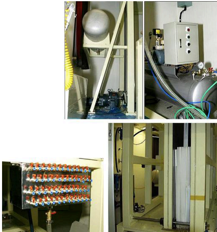
Figure 8: The oil coating facility
