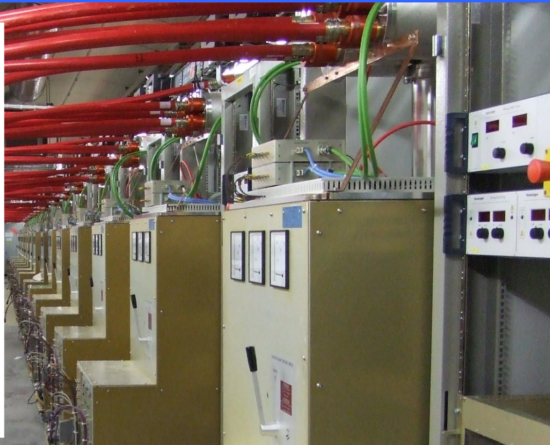
GTO stack with trigger transformer (right)
