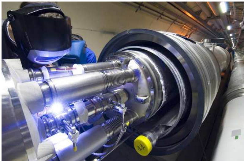
Figure 3.3: Photograph of one of the first LHC dipole magnets being installed in the LHC ring. From [39].
