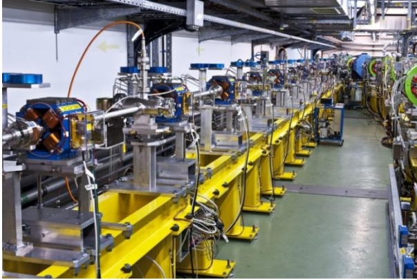
profile of the decelerated beam [5]. Figure 1 shows a photo of the TBL line installed in CTF3.
