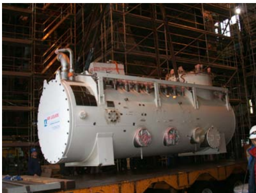
FIGURE 4. Cold box before lifting
