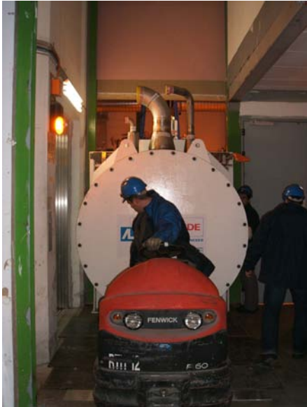
FIGURE 6. Cold box towing by tractor
