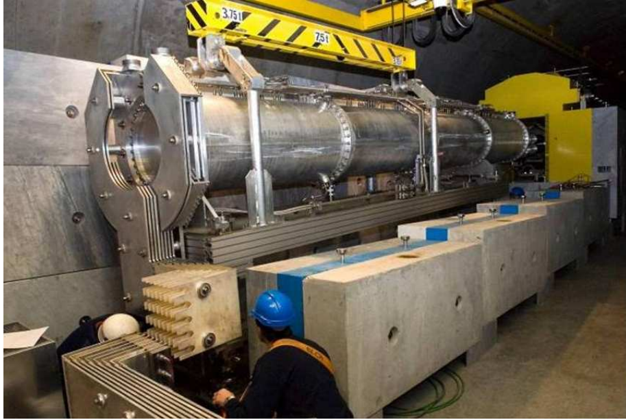
Figure 6. The CNGS horn during installation.
