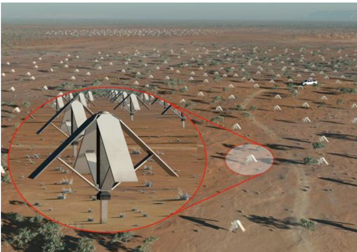
Figure 1: The SKA 1 concept involves two main receptor types, sparse aperture arrays (above, courtesy of Swinburne Astronomy Productions with enhancements by MAG) & dishes (see Fig.4).
