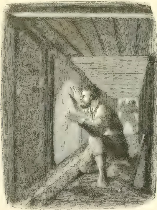
GALLERY AT SOUTH-EAST CORNER OF SANCTUARY.
