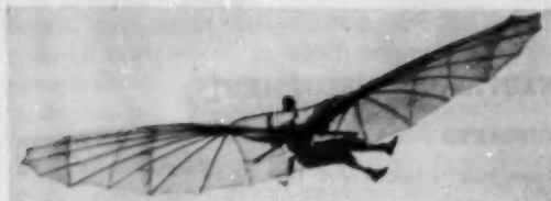
FIG. 1. Lilienthal got lateral control by shifting his weight.
