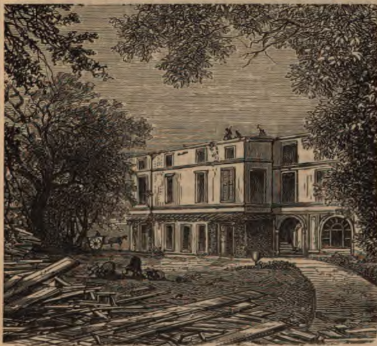
HOUSE OF M. THIERS DURING DEMOLITION AND REMOVAL.*
