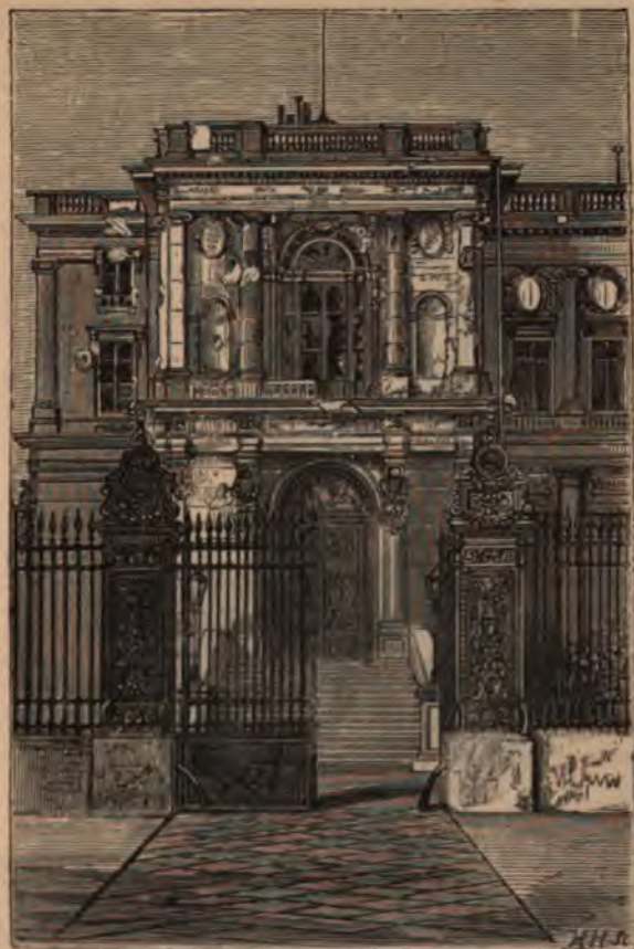
FOREIGN OFFICE (MUCH DAMAGED).
