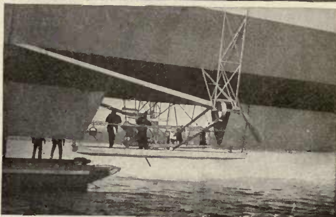
THE LZ. 6 (1908-10). IN THE LOWER RIGHT-HAND CORNER THE THIRD ENGINE INSTALLED AMIDSHIPS.
