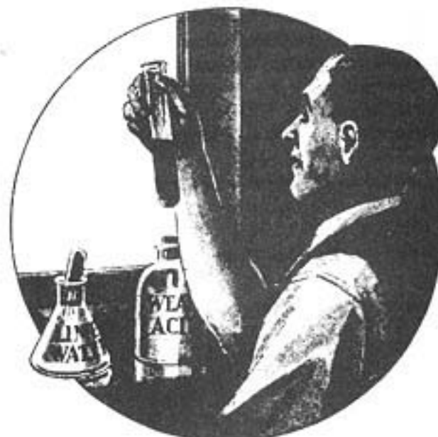
The dye solution used in testing soil for acidity or alkalinity should be made neutral by adding limewater or a weak acid solution, as needed, until it takes on the characteristic dark-green hue
