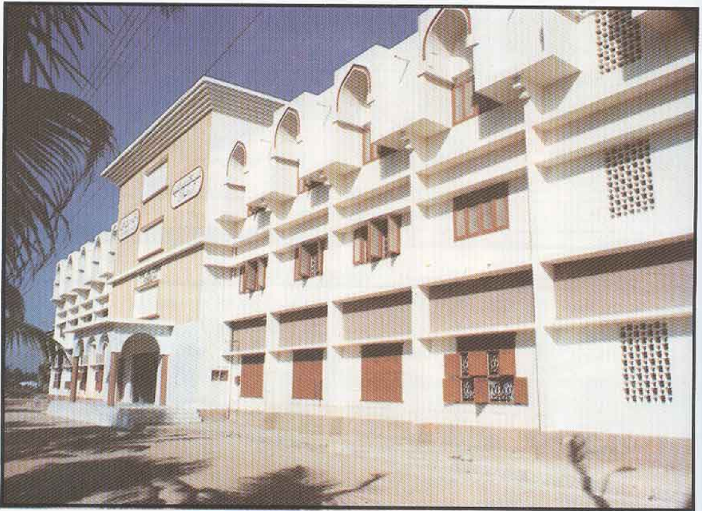
Primary and Secondary School building - front elevation.
