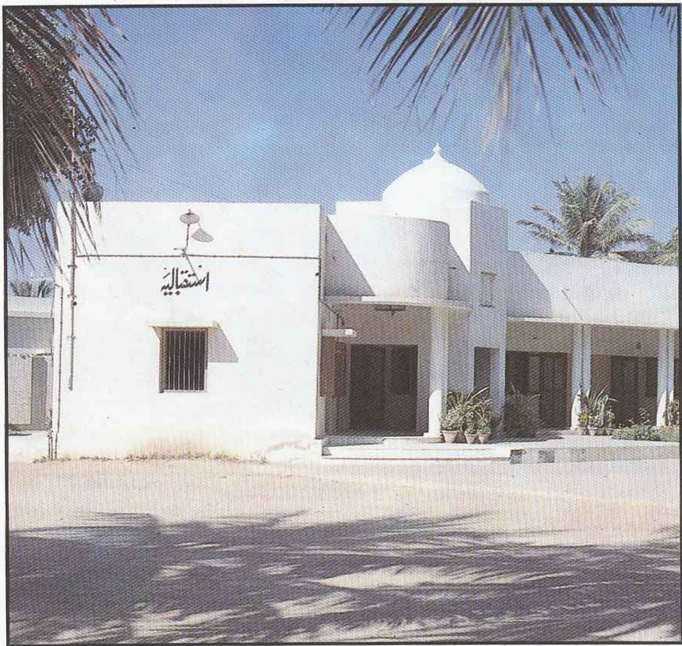
Reception, Telephone Switchboard and other Managerial Offices
