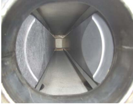
Figure 4: Photograph of the downstream end of the collimator prototype after it was hit repeatedly by a 2 MJ beam, up to 5 mm from the jaw edge. The left jaw (structured surface) is CC and the right jaw simple Graphite.
