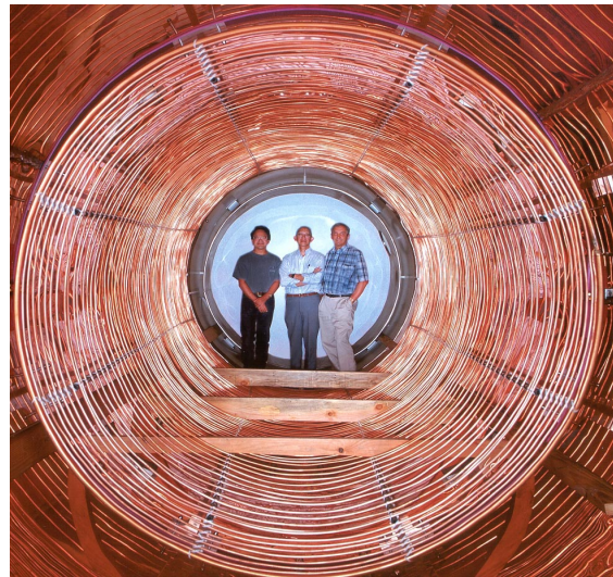
Figure 3: The air-coupled transformer primary
