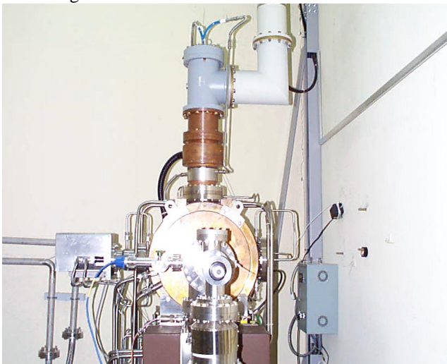
Figure 1. Prototype input coupler installed for the high power test.
