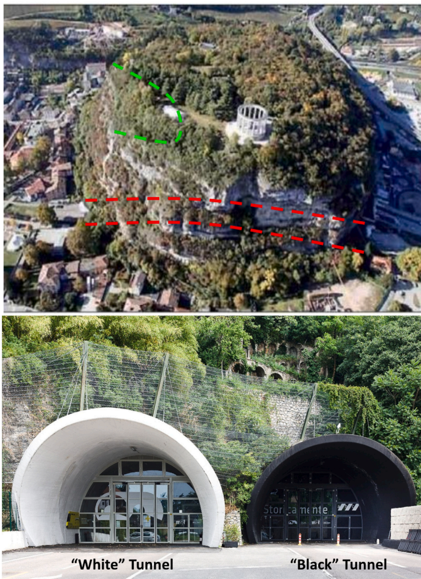
Fig. 1. The aerial view of the Doss Trento hill, embedded within the Piedicastello district near the Trento train station. Red dashed lines show the underground path of the two Piedicastello (White and Black) tunnels, while the green dashed line shows the path of the old tunnel crossed by the Alpini road.
