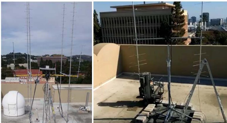
Figure 17. Left: UCLA's Knudsen North station with four UHF yagi antennas (downlink) and two VHF yagis (uplink, using power 10W). The spacing between UHF antennas is 6 feet on each side, and the spacing between VHF antennas is 10 feet. Right: Knudsen South station is a two VHF yagi providing higher output power (100W). Both stations can be used simultaneously and provide flexibility when both ELFIN satellites are within view.
