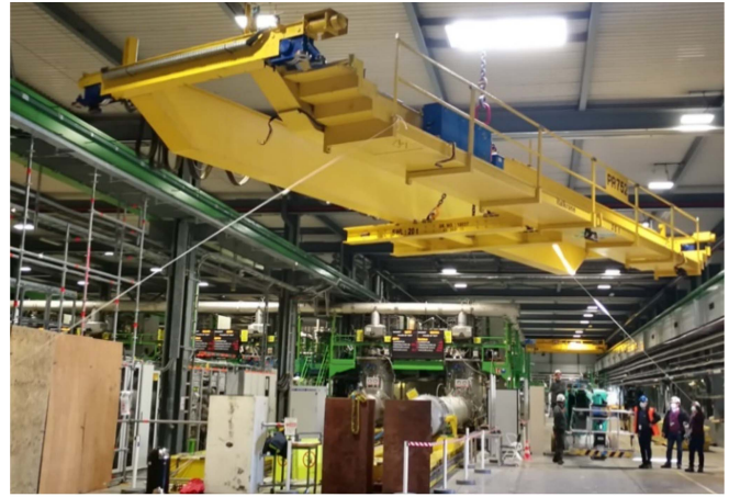
Fig. 2. Overhead crane being installed in SM18 building.
