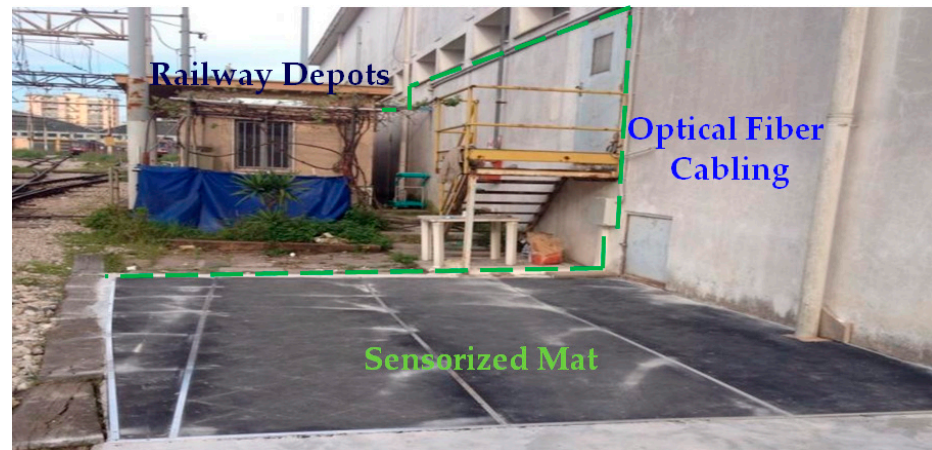
Figure 21. Intrusion detection system in a railway asset installed at the entry point of the Ponticelli depot. Reproduced with permission from ref. [161] (the figure is released under a Copyright Clearance Center's RightsLink® service).
